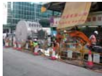
Equipment Set-up at Apliu Street
