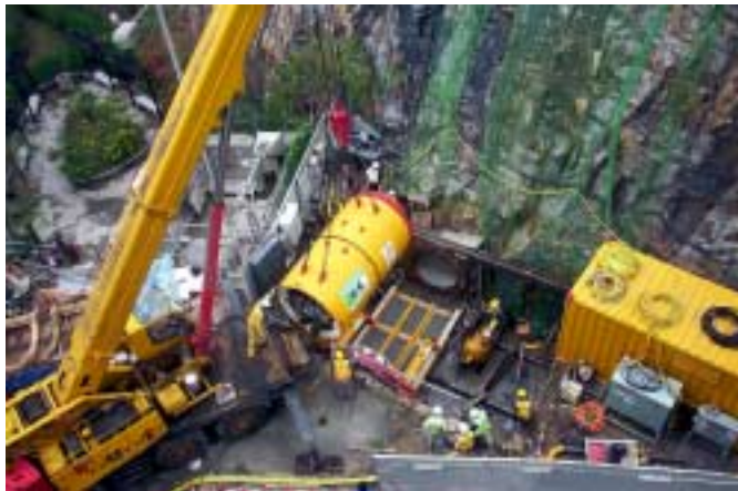
Placing the AVN1800T into the jacking pit.
